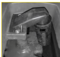
污水箱内水满保护装置 Sewage equips with full water device
